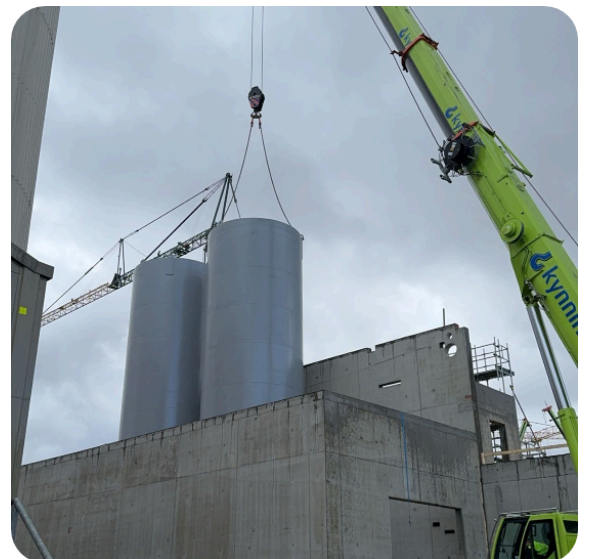
Sludge reception tanks delivered at Øra in Fredrikstad, Norway
