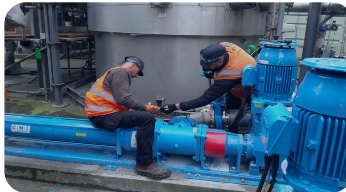
Pump upgrade at Davyhulme, Manchester, UK
