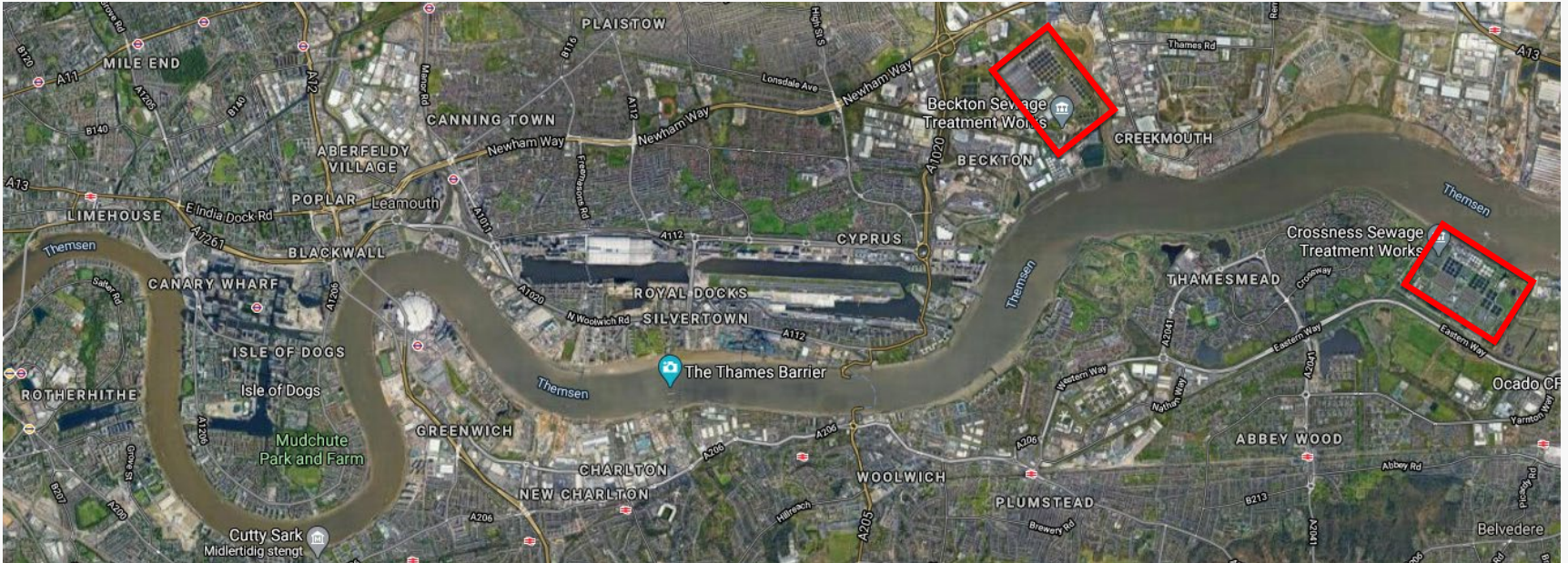
London map with Beckton (1864) and Crossness (1865) sewage treatment plants now located inside the city
