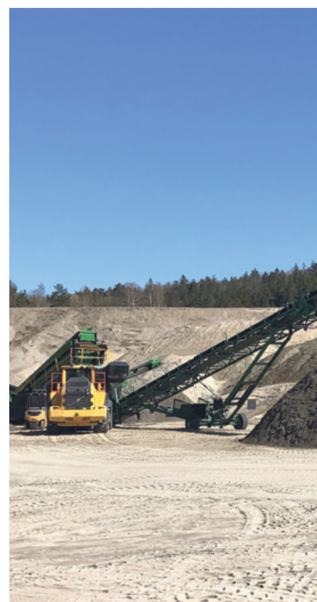
Reddal Sand soil production facility, Grimstad
